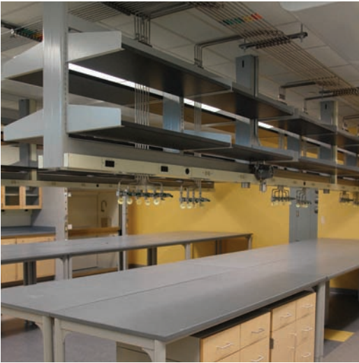
Suspended Overhead Carriers with adjustable shelving, electrical raceways, data outlets and service fixtures.
